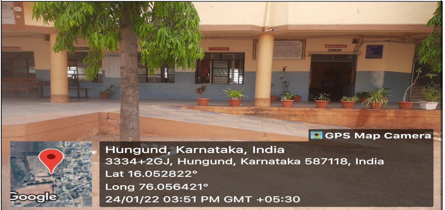
Ramp at office room
