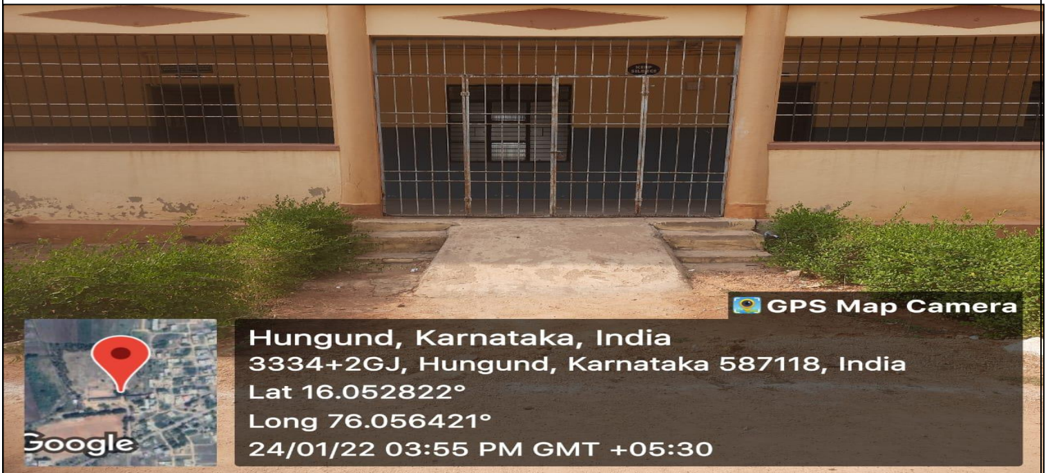
Ramp at class rooms
