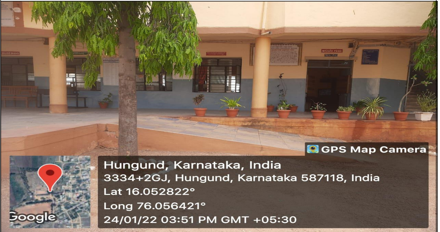
Ramp at the office building
