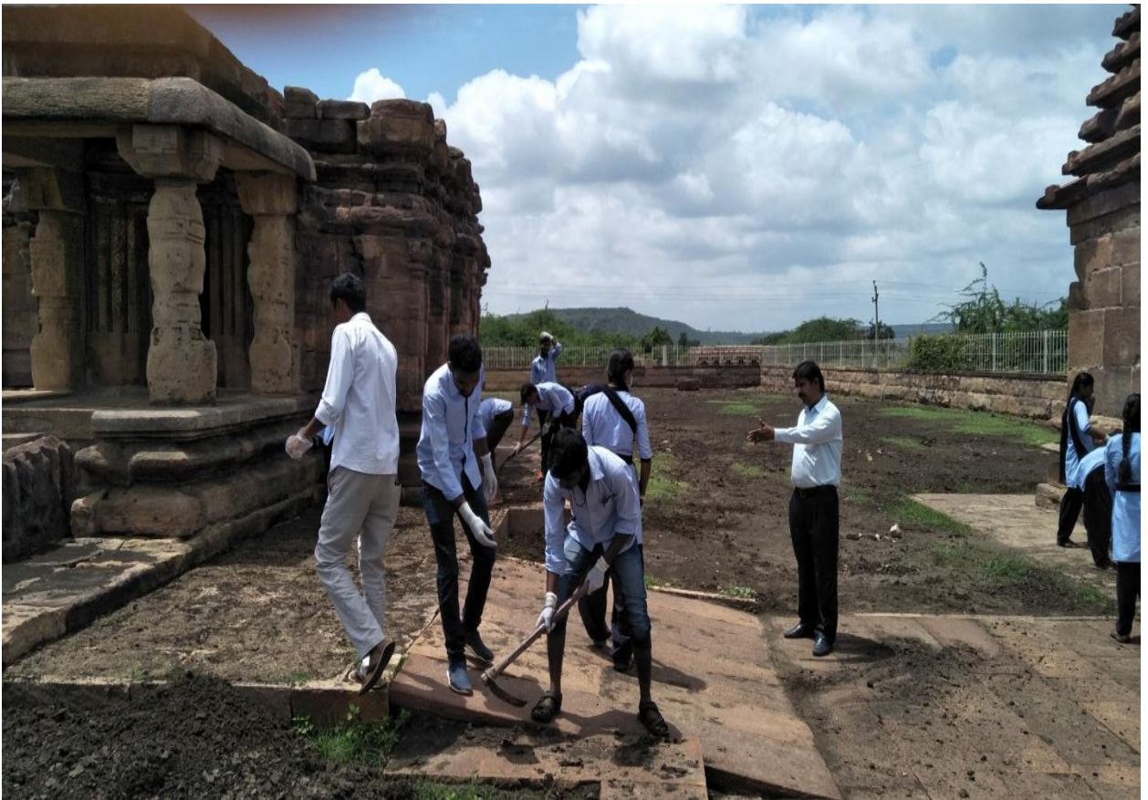
Students involved in Restoration of monuments from flood hit area
